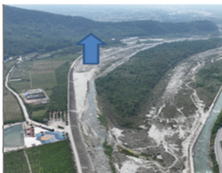
Figure 4. Suspected unfinished work
