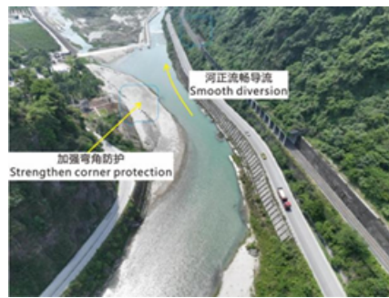
Figure 3. A realistic view of strengthening bay corner protection and smooth river diversion in the Luoshui project
