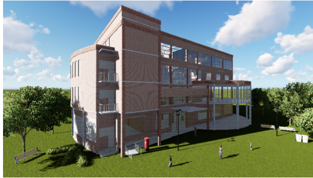
Figure 5. The east wall of the building.
