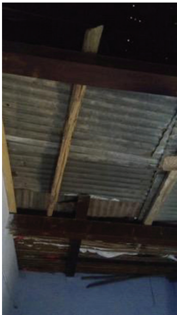
Figure 12. View of cement corrugated sheet added as false ceiling.
