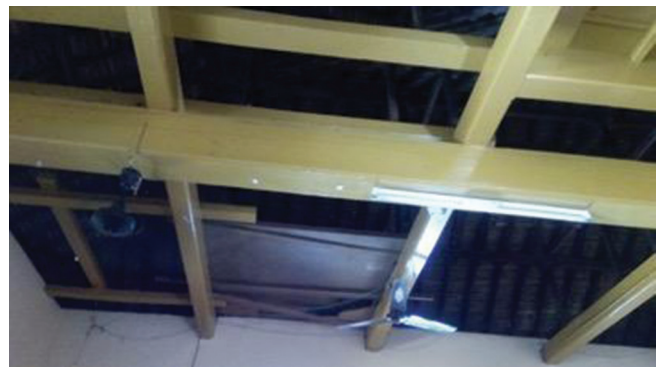
Figure 8. View of the main roof rafters.
