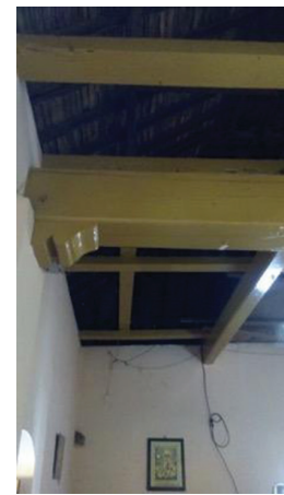
Figure 14. View of the main roof support system.
