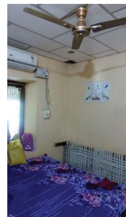
Figure 15. View of the false ceiling done in bedroom to avoid dust falling from the roof and air conditioner added for thermal comfort.
