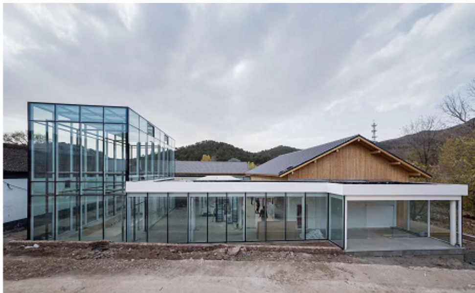
Figure 2. A photo of the Tmall Salon (under construction)
