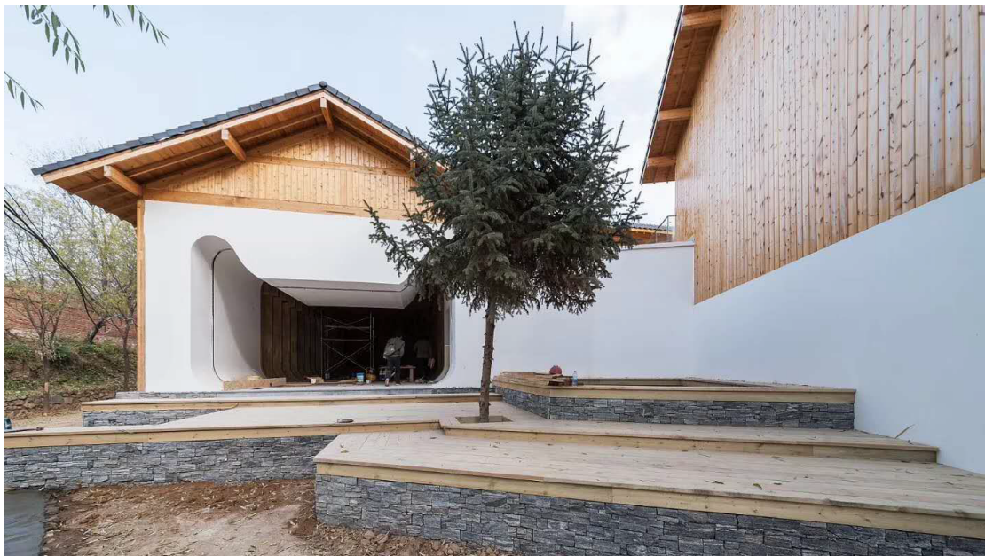
Figure 3. Main entrance to the Tmall Salon (under construction)
