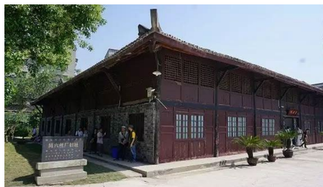
Figure 2. Liuhe Silk Factory Office Building. Source: Li Zhiming
