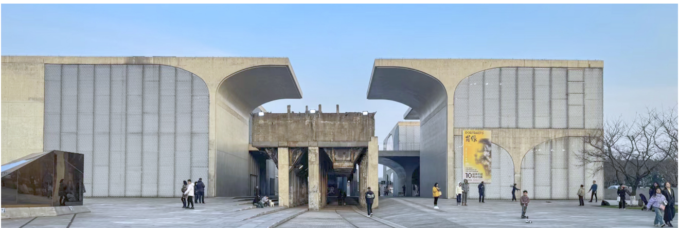
Figure 2. Southeast façade (Source: Author's picture)
