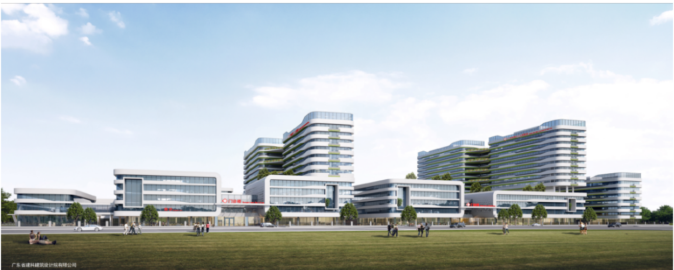
Figure 1. The new 12th People's Hospital of Guangzhou branch
