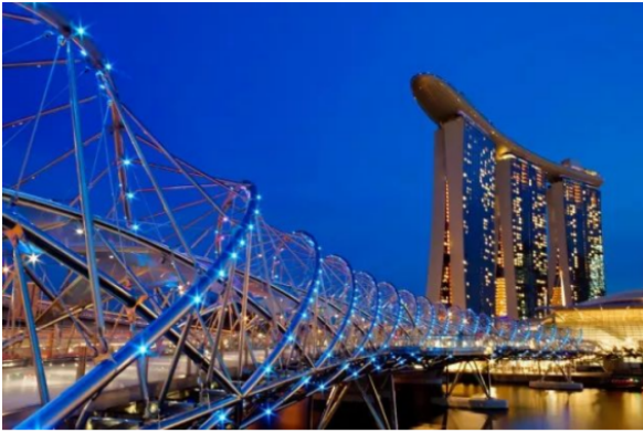
Figure 3. Singapore's Double Helix Bridge 1
