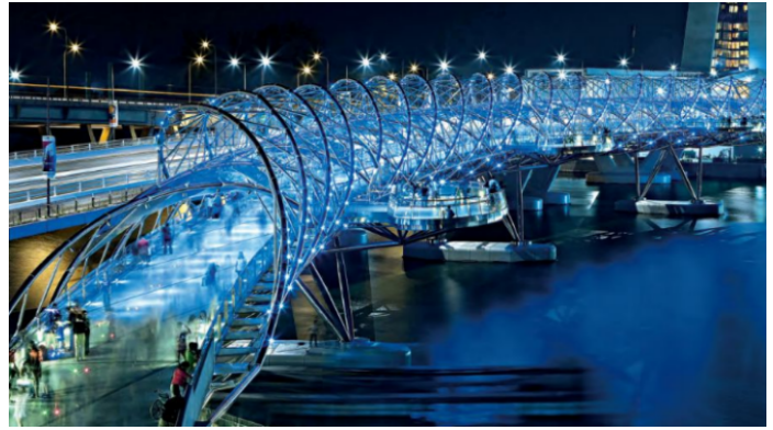
Figure 4. Singapore's Double Helix Bridge 2
