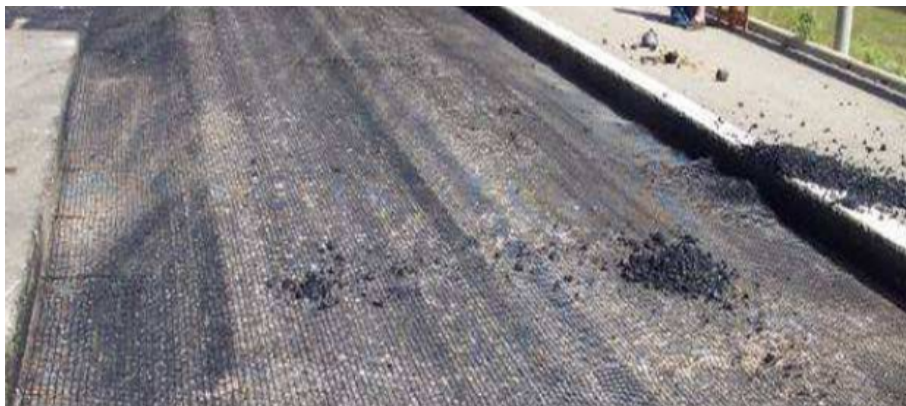
Figure 1. Schematic diagram of geogrid laying on roadbed
