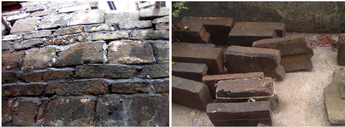
Figure 7. Bricks from the Han Dynasty in the walls. Source: photographed by Yuhua Zhu
