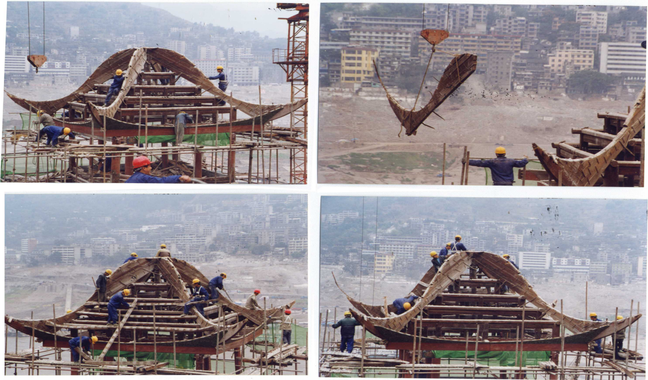
Figure 4. The helmet-shaped roof structure. Source: photographed by Yuhua Zhu
