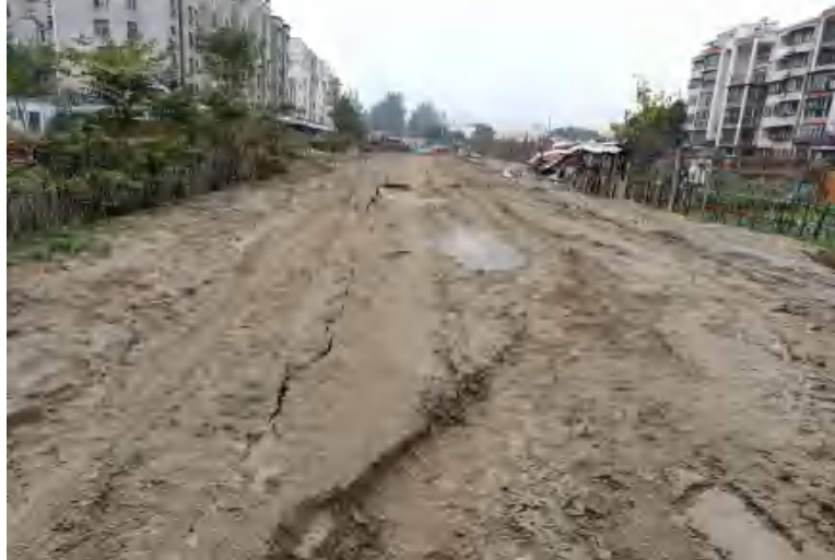
Figure 4. Collapse and grouting
