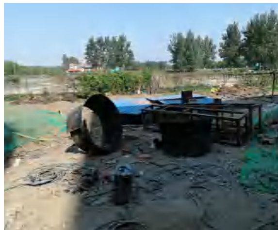
Figure 10. Sandbar pipeline dragging terminal elevation control device
