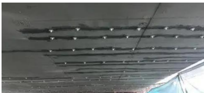
Figure 2. Bridge crack repair
