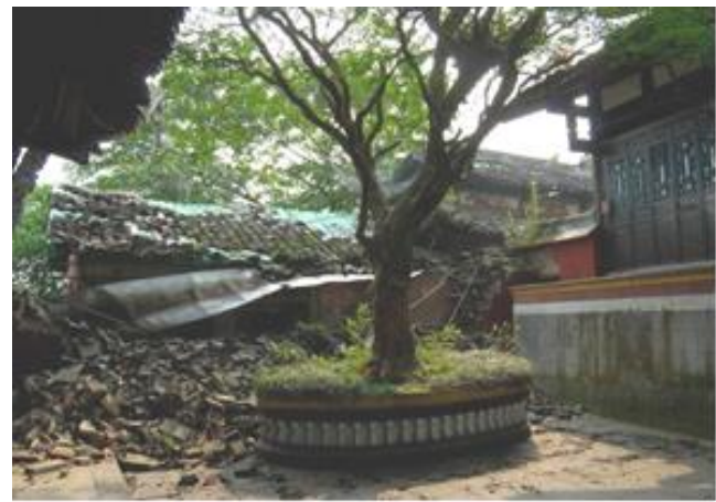
Figure 8. Front yard of Tiefo Hall after the earthquake
