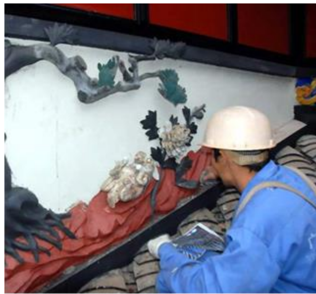
Figure 10. Conservation of decorations on the roof ridge
