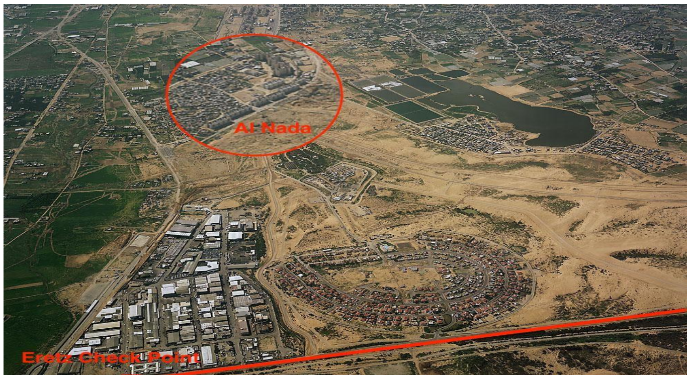
Figure 1. Aerial view of Al Nada right before the Israeli colonies demolition of 2008
