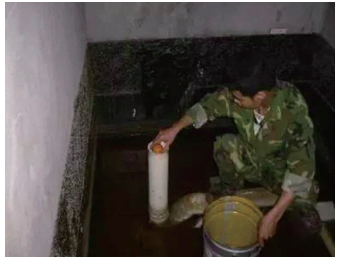
Figure 2. Sectional Inspection of Pipeline Irrigation
