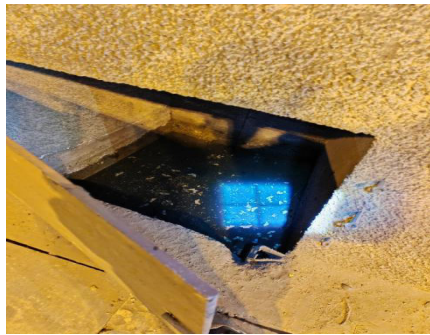
(c) Inspection of well water accumulation
