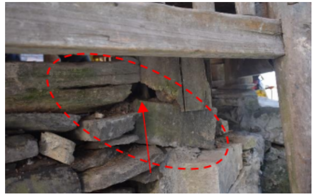
(b) Biological degradation at column bases
