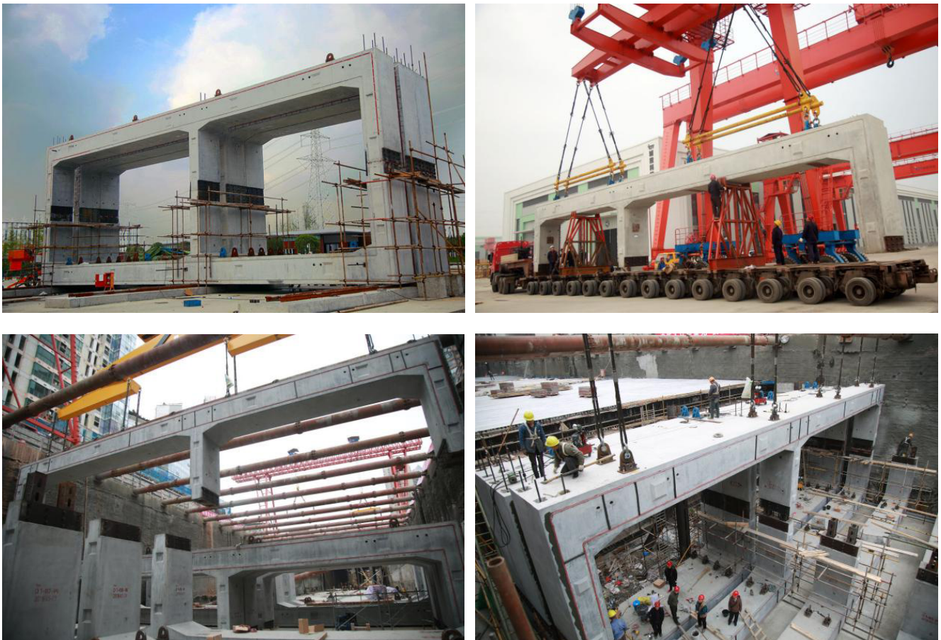
Figure 2. Photos of transportation and assembly of prefabricated components
