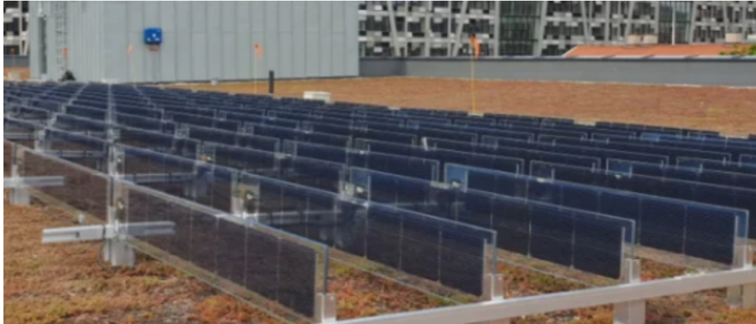
Figure 1. Small-scale experiment of rooftop HJT vertical power generation in Norway (Source: OverEasySolarAS)
