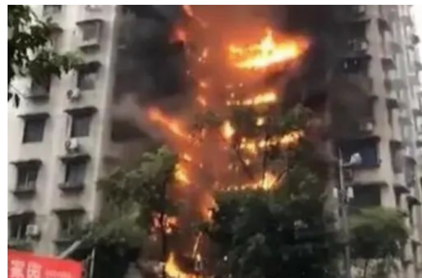
Figure 4. Photo of the fire
