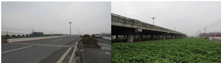
Figure 6. Actual photo of the Maqiao public-rail overpass.
