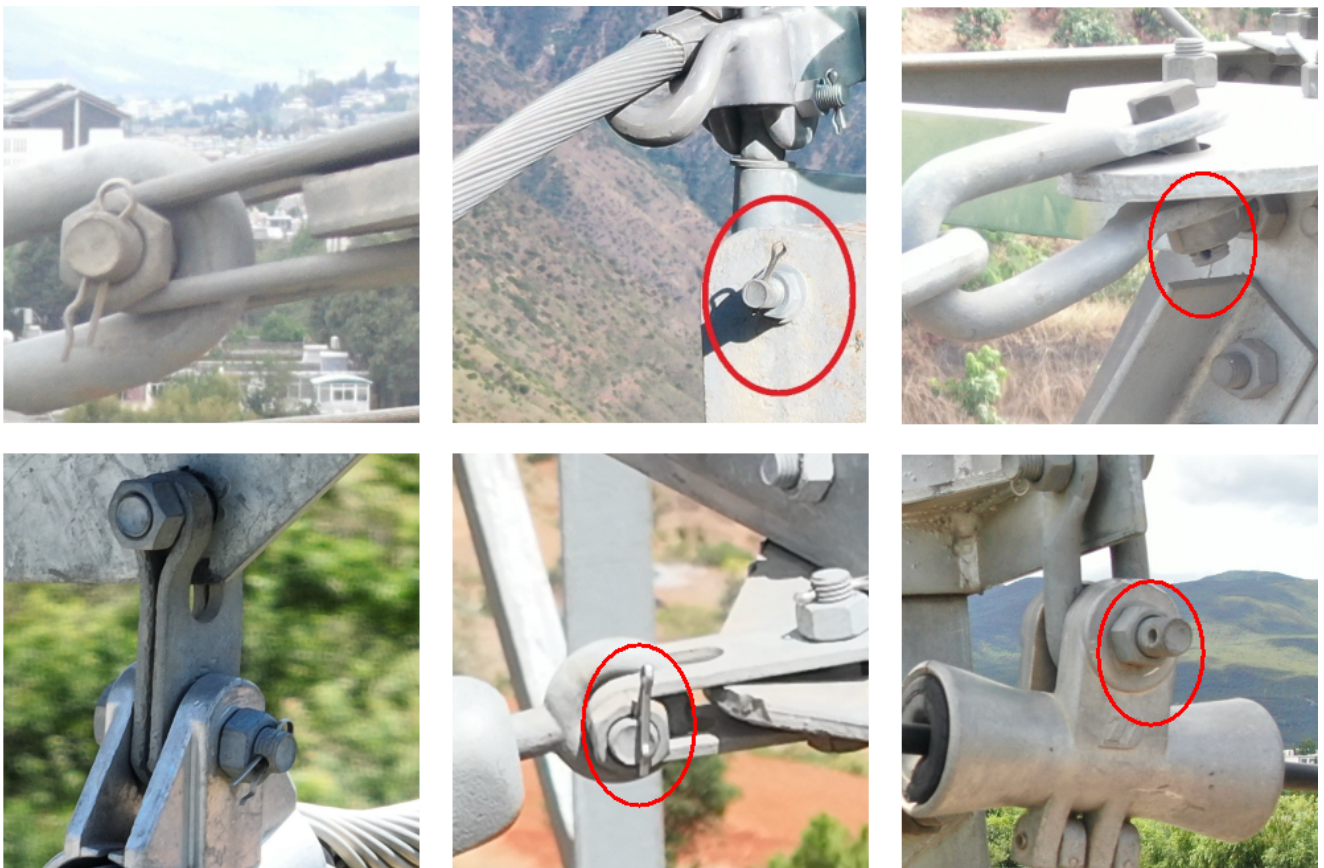
Figure 1. Schematic diagram of pin defects
