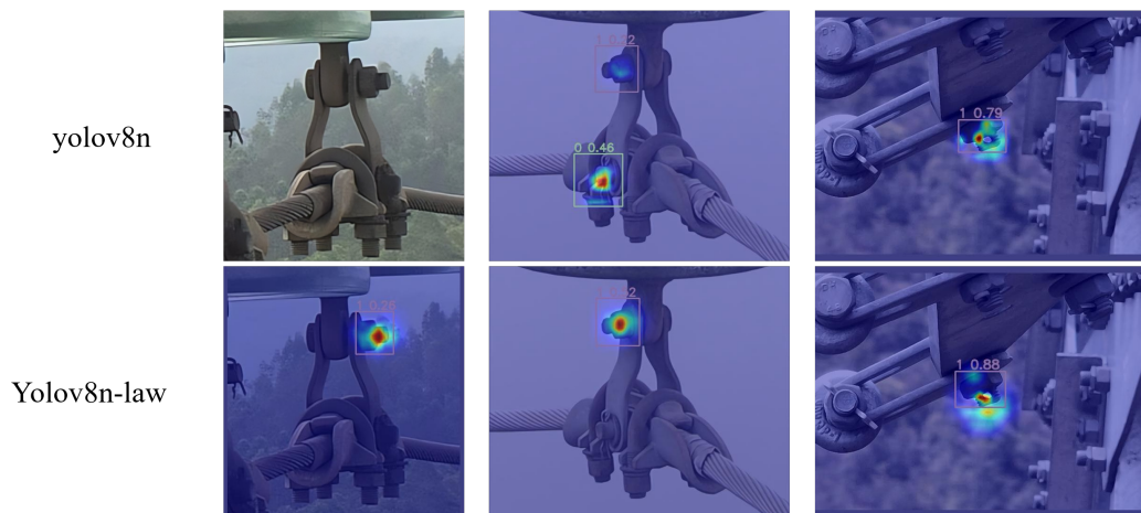
Figure 8. Heat maps comparing YOLOv8n and YOLOv8n-LWA (“0” and “1” denote the two defect types: abnormal pin and missing pin)
