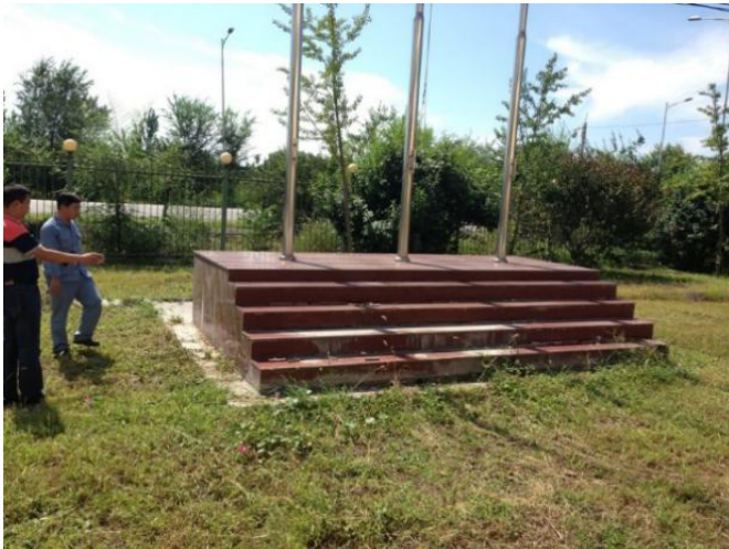
Figure 1. Pipe overlaid flag stand
