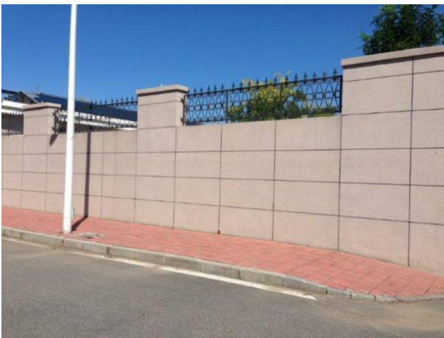
Figure 4. Brick wall on the pipeline
