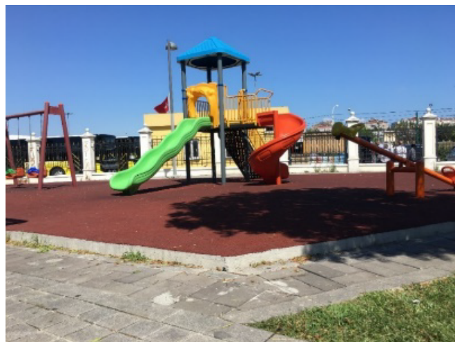
Figure 15. Zone 1, entrance to children's playground without ramp (Photo 12)
