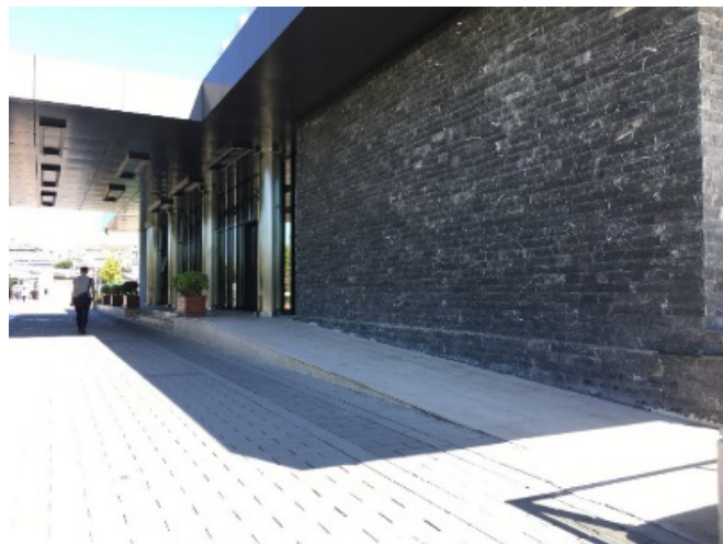
Figure 14. Zone 1, pavement ramp within the gardens (Photo 11)
