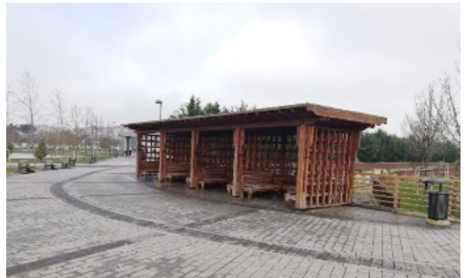
Figure 41. Zone 1, overhead elements 2 (Photo 37)
