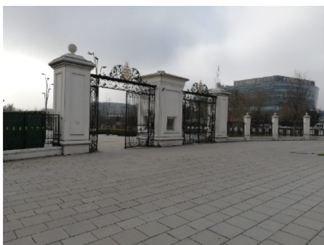
Figure 5. Zone 1, Entrance 2 (Photo 2)
