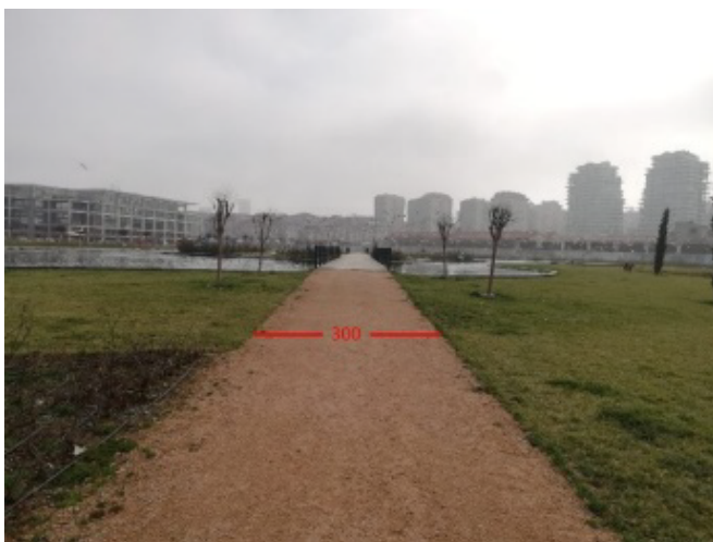
Figure 61. Zone 3, sloping pedestrian road (Photo 1)
