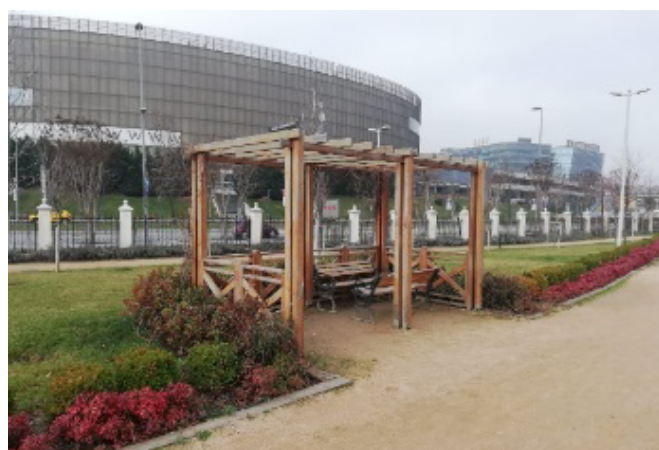
Figure 59. Zone 2, overhead cover elements and seating area (Photo 14)
