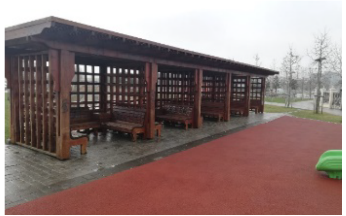
Figure 40. Zone 1, overhead elements 1 (Photo 36)
