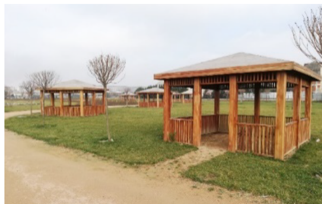
Figure 65. Zone 3, overhead protective elements (Photo 5)
