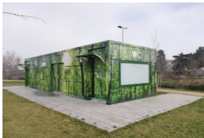
Figure 58. Zone 2, toilets (Photo 8)
