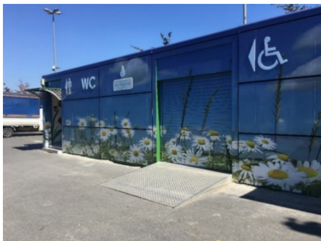
Figure 13. Zone 1, toilet ramp within the gardens (Photo 10)
