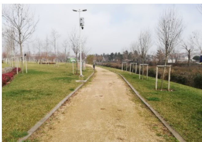
Figure 57. Zone 2, lighting elements (Photo 13)
