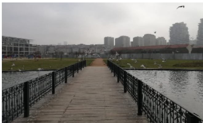
Figure 63. Zone 3, causeway over a lake (Photo 3)
