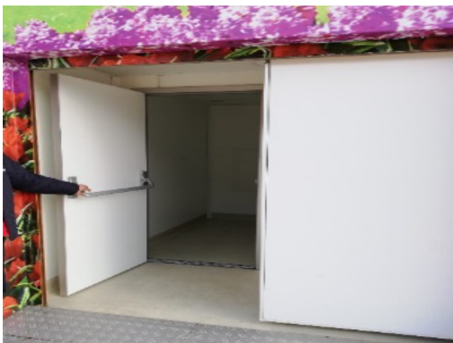
Figure 51. Zone 2, ramp (Photo 8)
