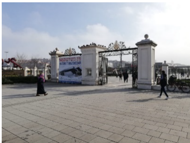
Figure 4. Zone 1 Entrance 1 (Photo 1)
