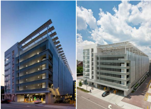
Figure 9. USA Green Square parking lot (Source: Construction Network)
