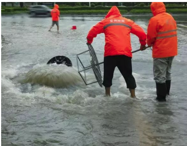
Figure 4. Rainwater from the middle and lower reaches emerges from the inspection wells and rainwater rafters
