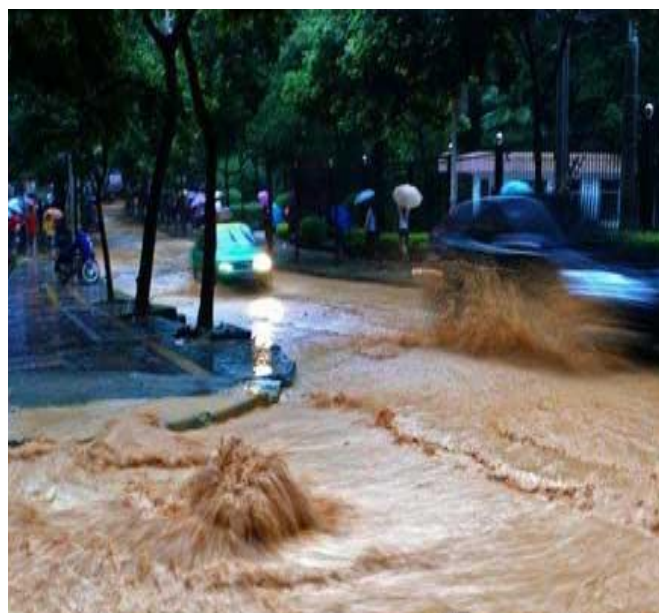
Figure 3. Slops emerging out of rainwater inspection well and gutter strainer due to upstream water pressure and water being pushed from downstream
