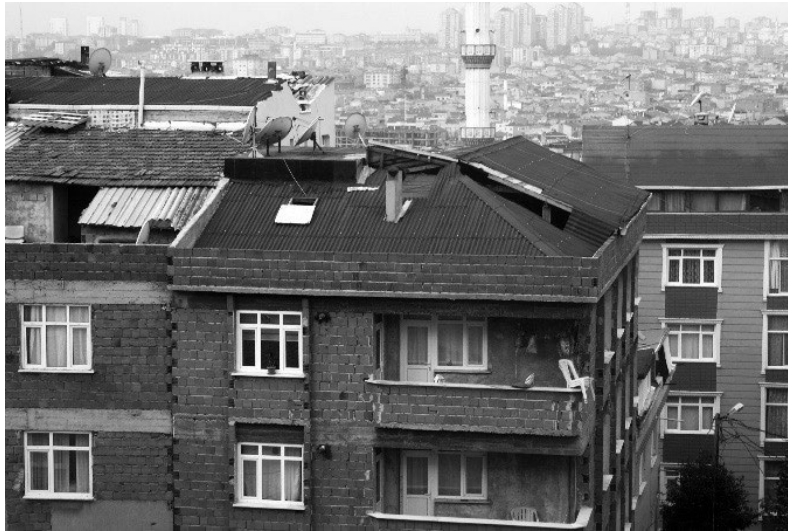
Figure 5. Rooftop in İstanbul, photographer Hüray Kazan, copyright holder Esen Gökçe Özdamar
