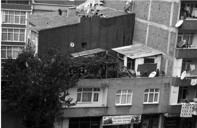
Figure 2. Rooftop in İstanbul, photographer Hüray Kazan, copyright holder Esen Gökçe Özdamar
