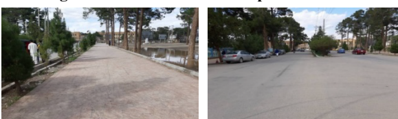
Figure 4. Left: Stone Masonry Pathways; right: Main roadways
