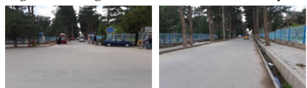
Figure 5. Left: East West Roadway; right: Northern Roadway
