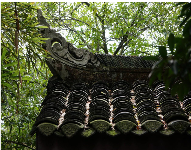
Figure 10. Dongpo Academy Ruyi cloud pattern main ridge (Source: Photographed by the author)
