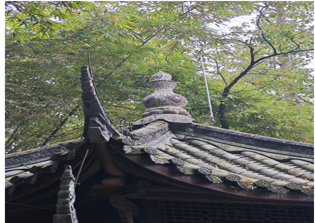
Figure 9. Baoyue Pavilion porcelain piece inlaid flower ridge spire (Source: Photographed by the author)
