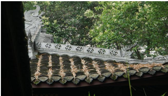
Figure 4. Lai Feng Pavilion “Thousand Character” pattern gray sculpted ridge decoration (Source: Photographed by the author)
