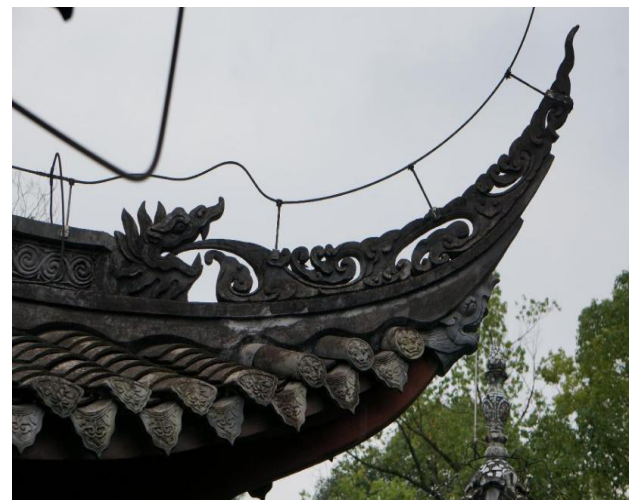
Figure 11. Baipo Pavilion Ruyi water pattern flying eaves (Source: Photographed by the author)
