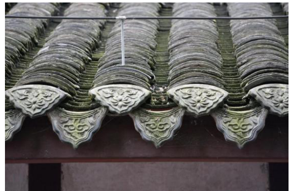
Figure 7. Lai Feng Pavilion Ruyi lotus pattern tile work (Source: Photographed by the author)
