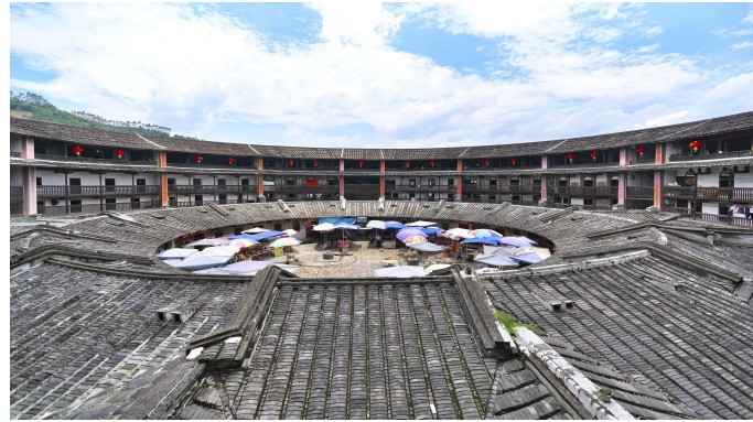
Figure 2. Er Yi Building in Hua an County (Source: https://pixabay.com/zh/ )
