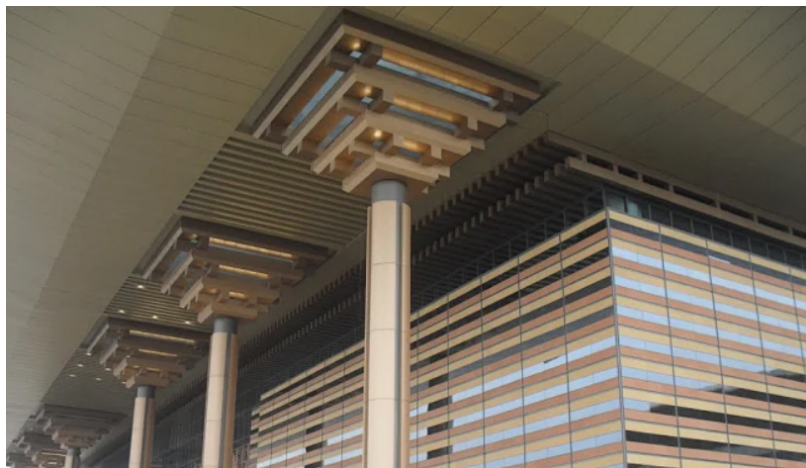
Figure 2. Photo of the Bracket Set elements at the entrance of Nanjing South Railway Station
