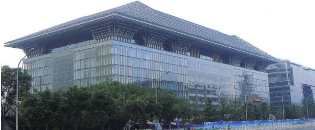
Figure 3. Photo of the China Development Bank office building
