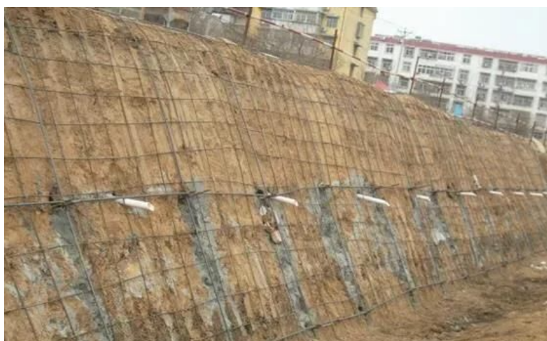
Figure 2. Soil nailing technology
