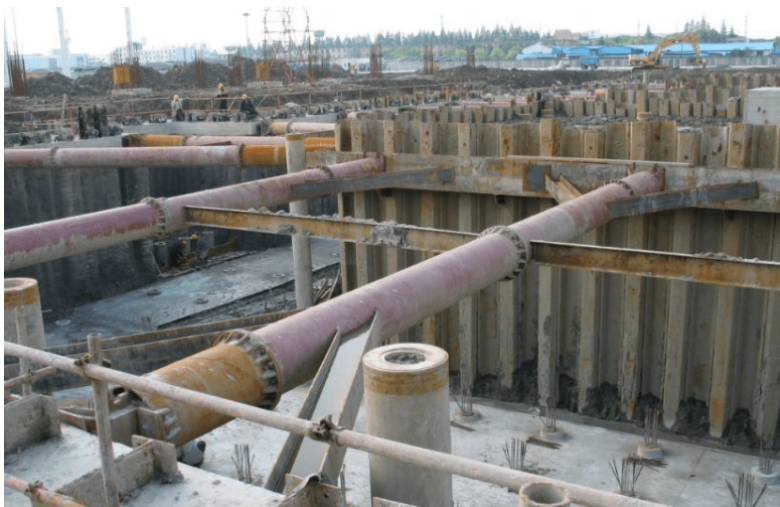
Figure 1. Row pile support technology
