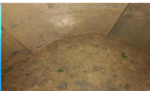
Figure 11. Soil sample at pile bottom
