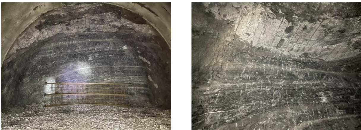
Figure 4. Photos of the surrounding rock conditions of ZK41+444 tunnel face
