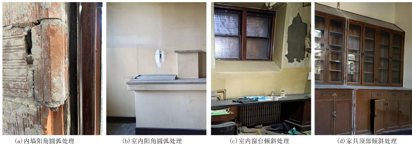
Figure 4. Indoor fillet treatment of Peking Union Medical College. (a) The circular arc treatment of the inner wall exposed corners. (b) Arc treatment of indoor exposed corners. (c) The sloped treatment of indoor windowsills. (d) Tilt treatment of furniture tops.
