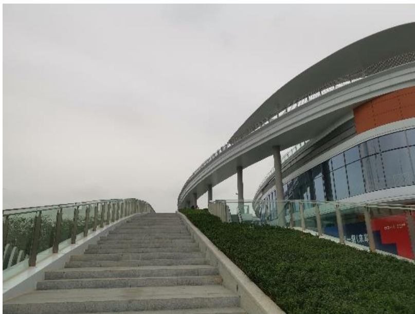
Figure 4. Roof of Happy Harbor
