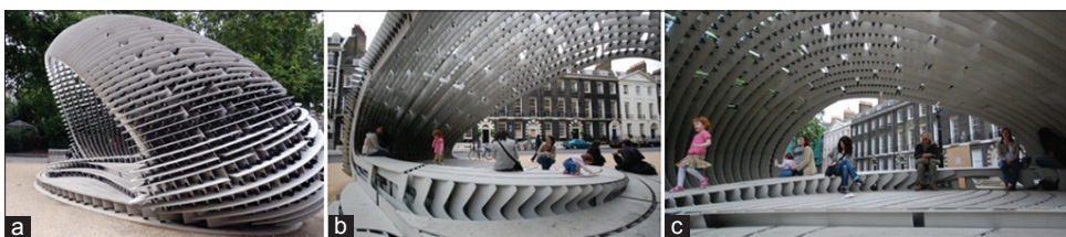
Figure 11. (a-c) Fiber-C, glass fiber-reinforced concrete material, Bedford Square, London, United Kingdom, Zaha Hadid Architects, Synthesis Design + Architecture w/Nex Architecture, Adams Kara Taylor [26]
