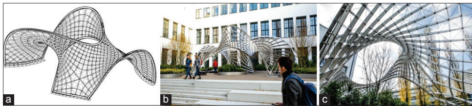
Figure 7. (a-c) Catenoid form, inside/out research pavilion at the central campus of the TUM, Munich [17]
