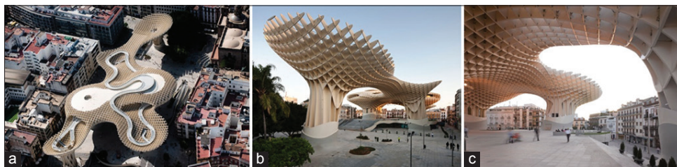
Figure 17. (a-c) The timber lattice system, Metropol Parasol Seville, Spain 2011 Jürgen Mayer H., 3400 individual wooden elements, 28.50 meters, concrete, timber and steel tree-shaped shading structure, high representation of free-form, prefabricated and assembled on-site, the freedom in making the node, or manufacturing the wood element [40,41]
