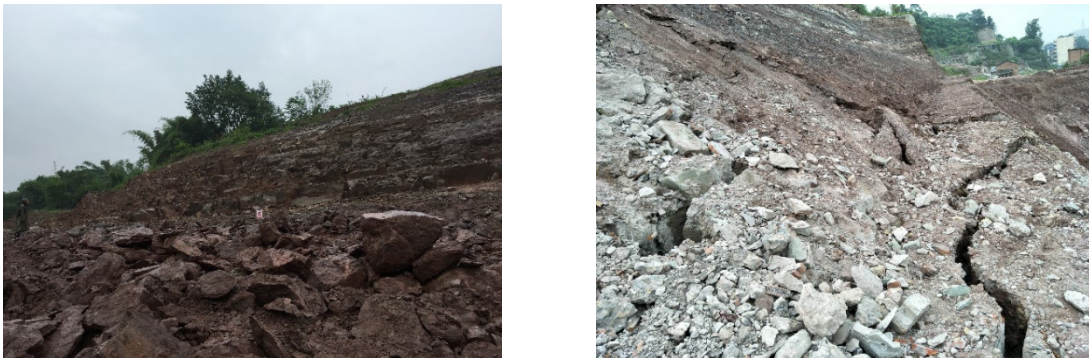
Figure 1. Photo of landslide during project construction
