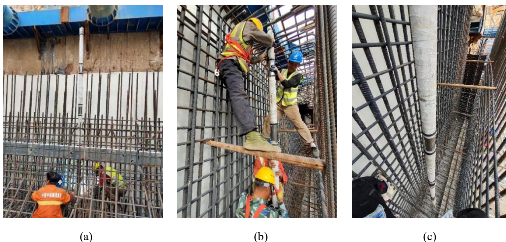
Figure 5. Installation of the embedded steel pipe
