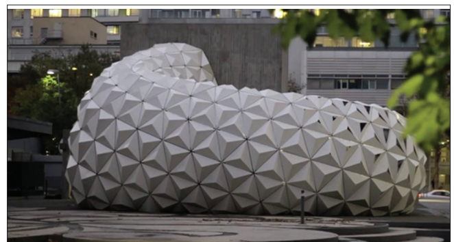
Figure 14. Arboskin pavilion by ITKE, Stuttgart, 2016 [43]
