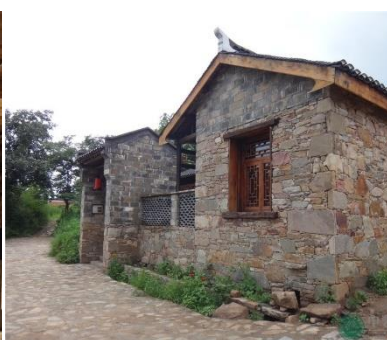
Figure 2. Renovation of Taoyuan village
