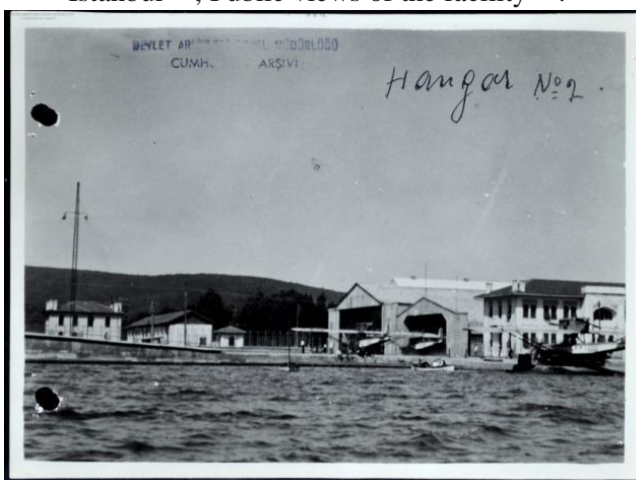
Figure 3. and Figure 4. AEI scaffolding, Istanbul [29] ; Public views of the facility [29] .
