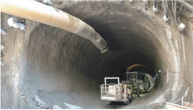
Fig.1 The Actual Shot of the Low-gas Tunnel Construction
