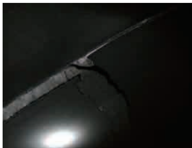
Figure 3. Faulting of slab ends on the secondary lining on the right side of vault of the k21+275 segments
