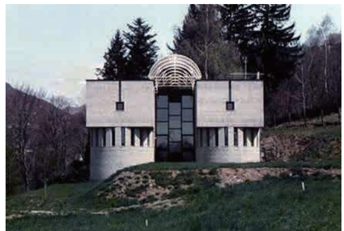
Figure 21. Mario Botta's house in Origgio [66] .
