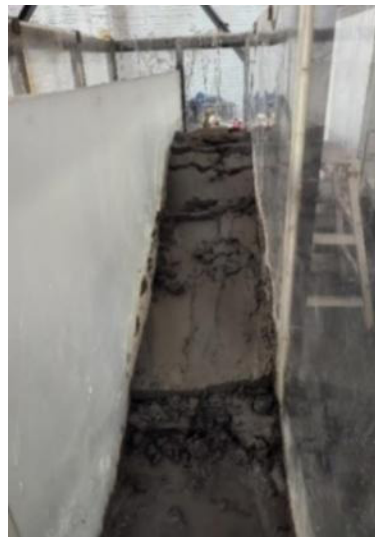
(a) Front view of tailings dam failure
