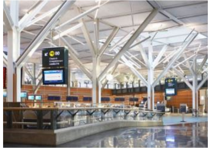
Figure 15. Frankfurt Airport Pillar Tree Form - pinterest.co.uk.
