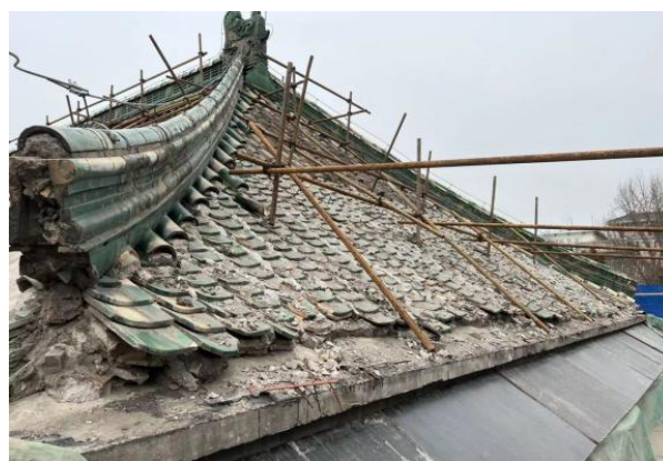
Figure 7. Roof waterproofing treatment
